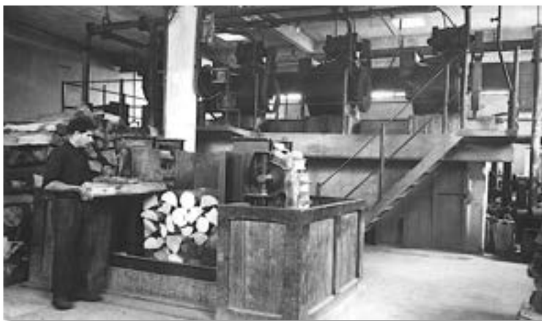
Chipper machine. Cartiere Meridionali. Four turbines can be seen behind.
