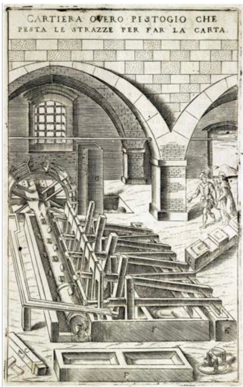
“Pistogio” for beating rags in the 18th century paper mill.
