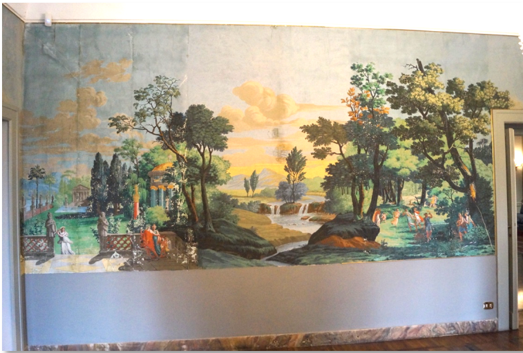
Wallpaper made with a 24-colour machine, of the type produced in the adjacent Fabbrica San Carlo. Image taken courtesy of the Nota family. Note on the left the partial lifting of the paper due to moisture infiltration.
