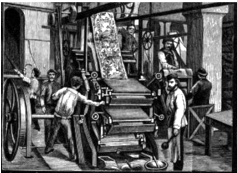
The “upper perspective part” or top part of the 24-colour machine.
