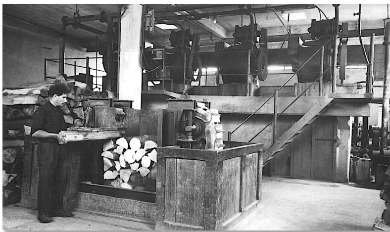
Chipper machine. Southern Paper Mills. Four turbines can be seen behind.
